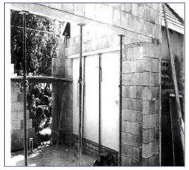
A & D Holdings external wall interlocking blocks
