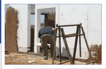
EPS Bygg external walls covered with mesh and plaster
