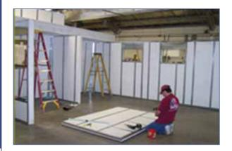
Ecodwell panel walls showing EPS core and lightweight steel framing
