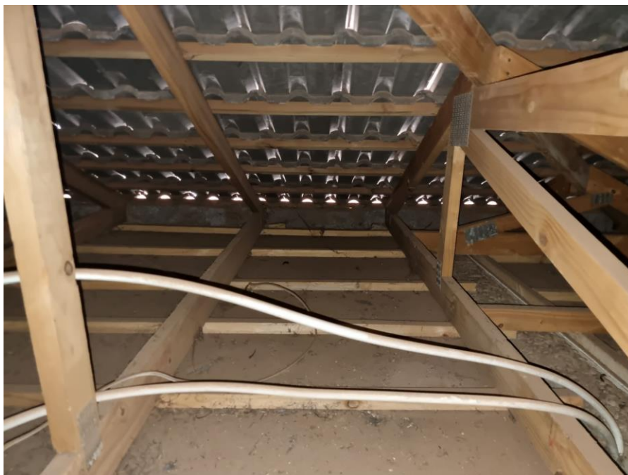
Figure 19: Double roman concrete roof tiles
