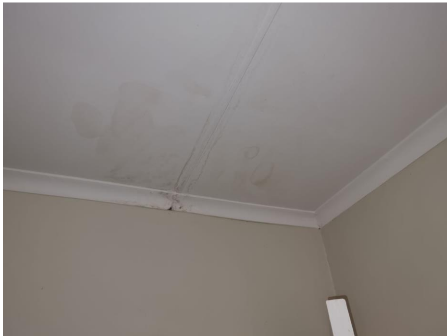
Figure 13: Ceiling and cornice
