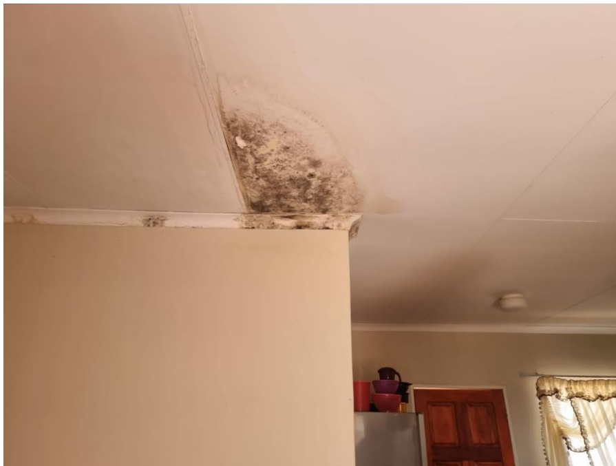
Figure 5: Ceiling and cornice
