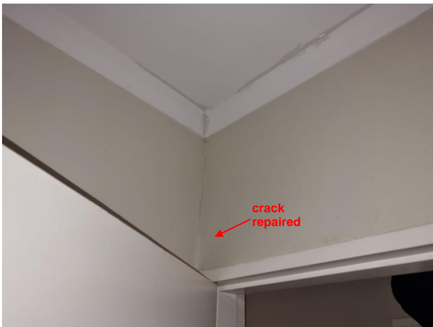
Figure 11: Ceiling and cornice
