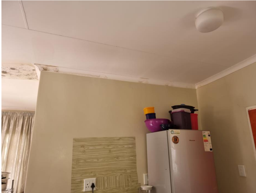
Figure 4: Ceiling and cornices
