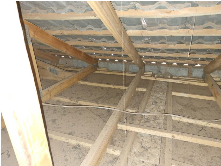
Figure 17: Engineered timber roof trusses and galvanised truss anchors
