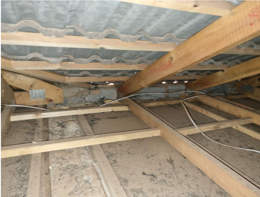
Figure 18: Galvanised truss anchors
