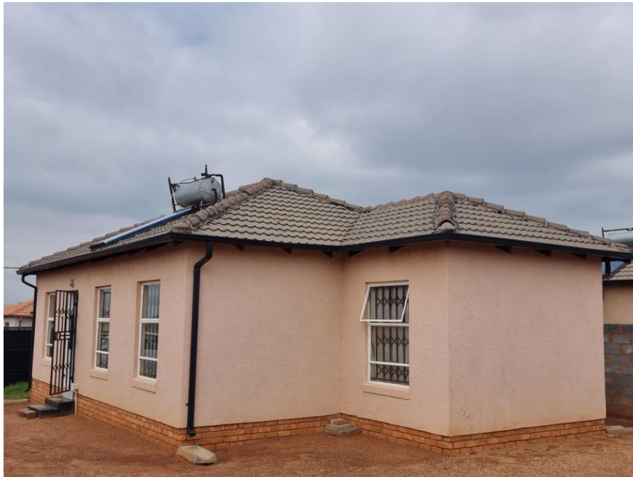
Figure 22: Rear/side elevation of the house
