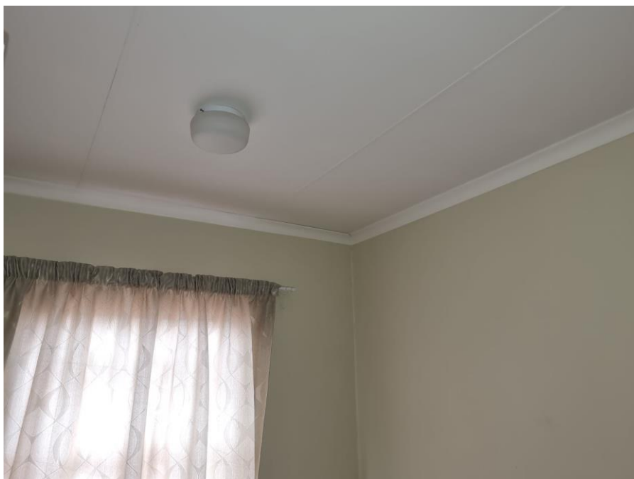
Figure 15: Ceiling and cornice
