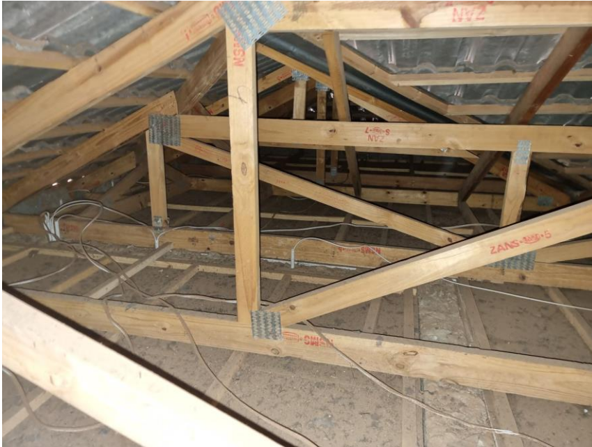
Figure 16: Engineered timber roof trusses with concrete tile covering
