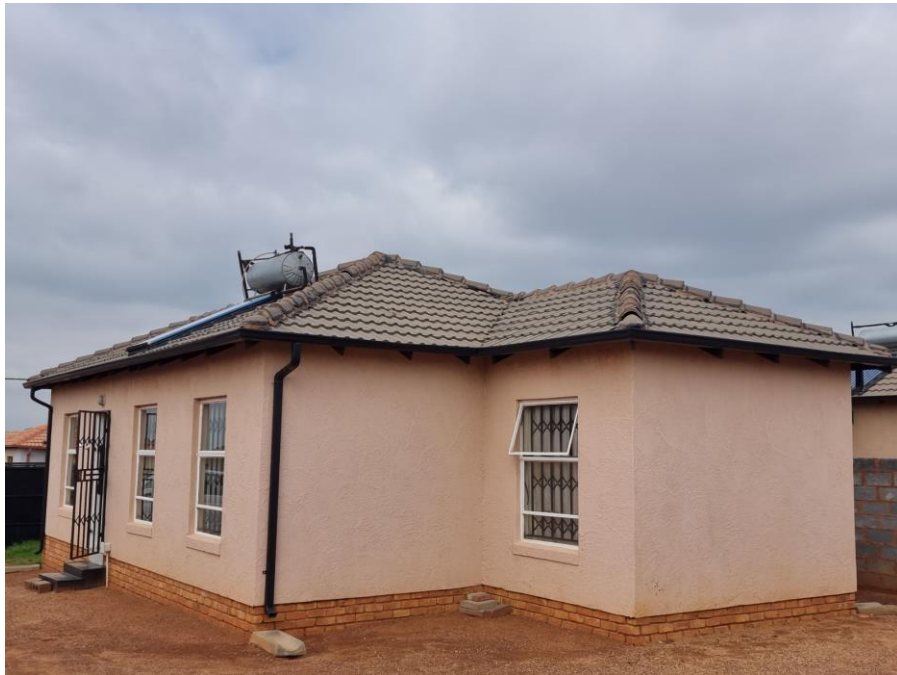
Figure 24: Rear/side elevation of the house
