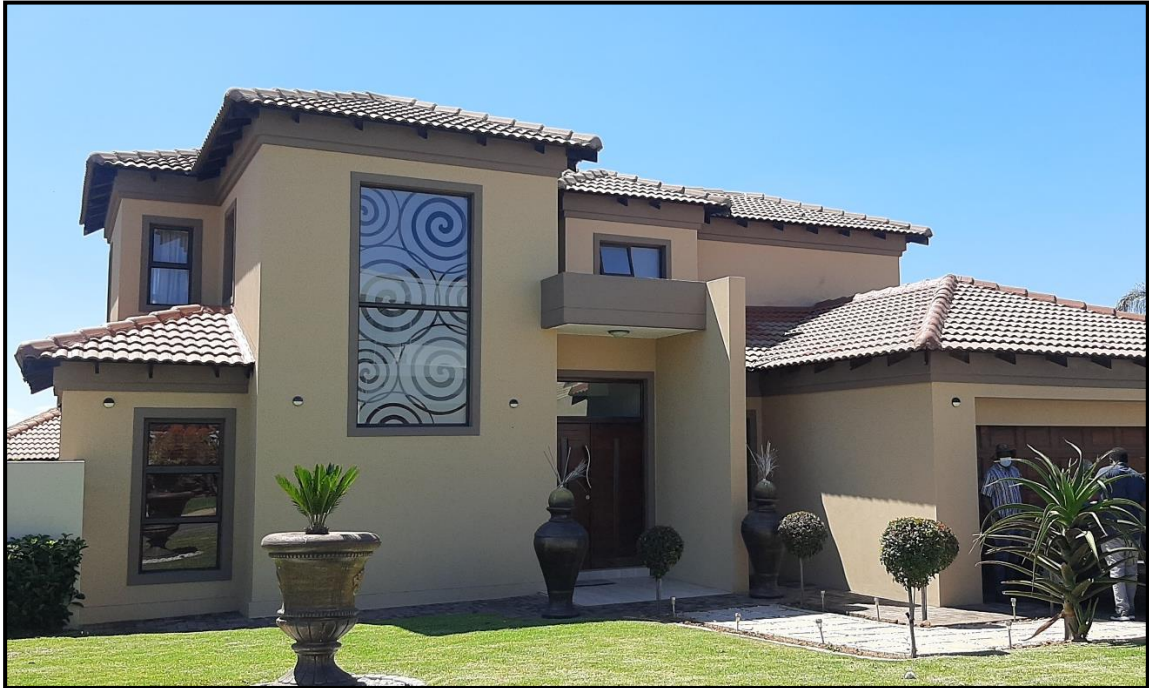
Figure 1-2 Building Elevation – House Mngadi (view from Street Entrance)
