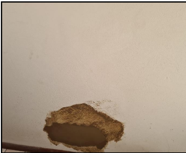
Figure 5-7 Sampling Popped Bricks - Image 02
