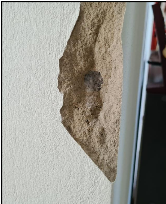
Figure 5-1 Brick pops – Pyjama Lounge – Image 01
