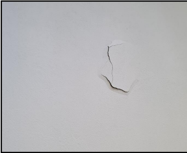
Figure 5-6 Sampling Popped Bricks - Image 01
