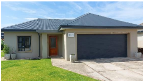
Pic 01: North Elevation of building
