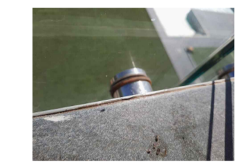
Water seeps into ceiling void in Living room
