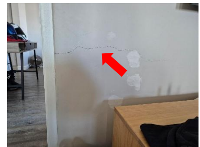
Pic 07: Crack in wall at Bedroom 3 door entrance
