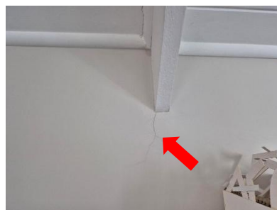
Pic 03: Crack at each support location of roof truss at wall plate level
