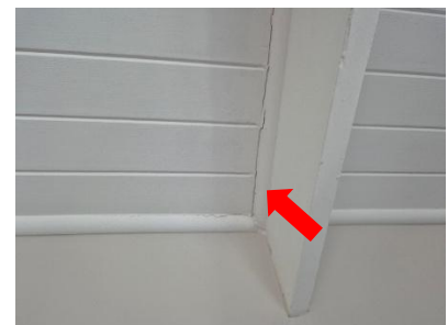
Pic 04: Separation of roof assembly finishing elements
