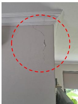
Pic 01: Vertical crack in wall
