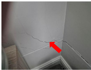
Pic 06: Crack in corner of bedroom 3 wall and above upstand beam level
