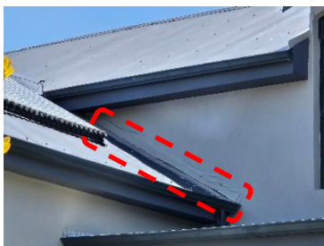
Pic 08: Defective roof flashing and water proofing
