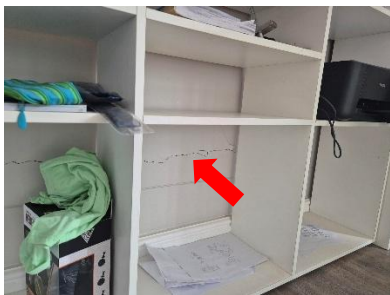
Pic 05: Horizontal crack above upstand beam level
