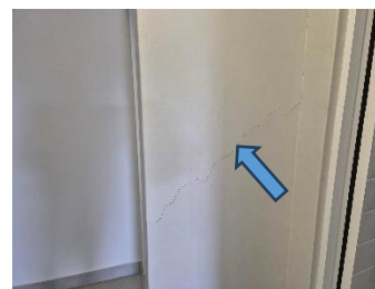
Pic 06: Diagonal crack in wall from settlement of surface bed.
