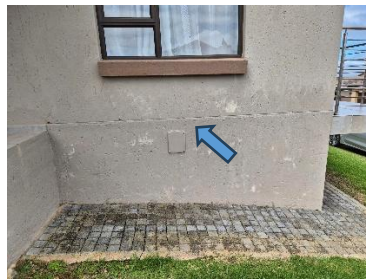
Pic 02: Settlement cracks above and below V-joint
