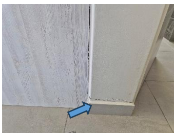
Pic 04: Settlement of internal wall and detach from cupboard.
