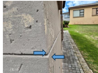
Pic 03: Outwards movement of foundation walls with cracks
