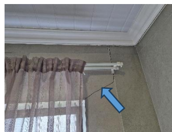
Pic 05: Large differential crack above window
