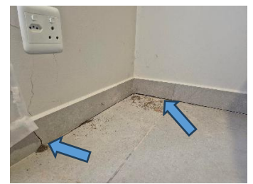
Pic 07: Settlement (>10mm) of surface bed and crack in wall.
