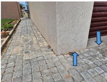
Pic 01: Paving level same as Garage FFL with no weepholes in walls.
