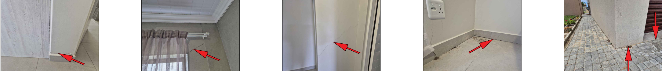
1 Settlement crack in internal wall 2 Differential crack above window 3 diagonal crack in internal dividing wall 4 Settlement of surface bed 5 Paving level same as garage FFL 6 Settlement crack below construction joint 7 Visible gaps between paving blocks, drain water 8 Foundation wall >1000mm with 1 x weep hole opening 9 Outer movement of foundation wall (undersailing) 10 Crack in foundation wall 11 Detached ceiling cornice - wall settlement 12 Separation crack in foundation wall 13 Cantilever concrete deck with cracks underneath
