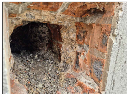
Picture 14 - Open section in wall indicating concrete filled 280 foundation wall
