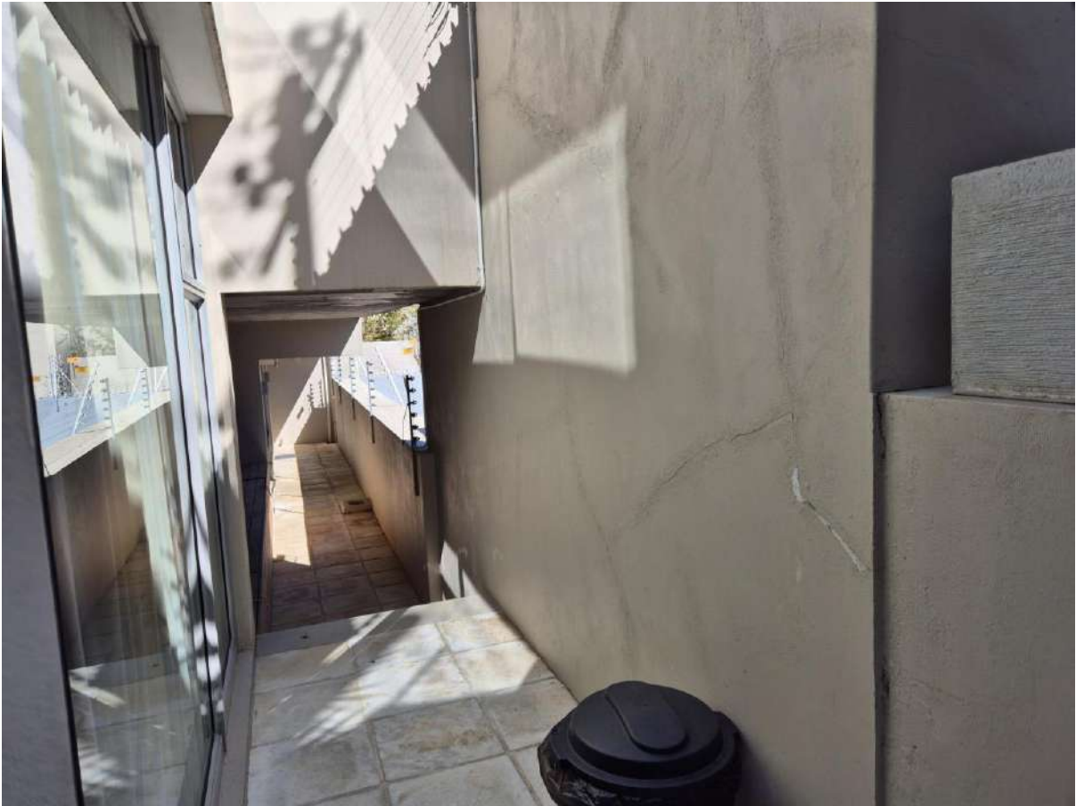
Wall area beneath the neighbor with the compromised and irregular roof structure and poor finished plaster work.
