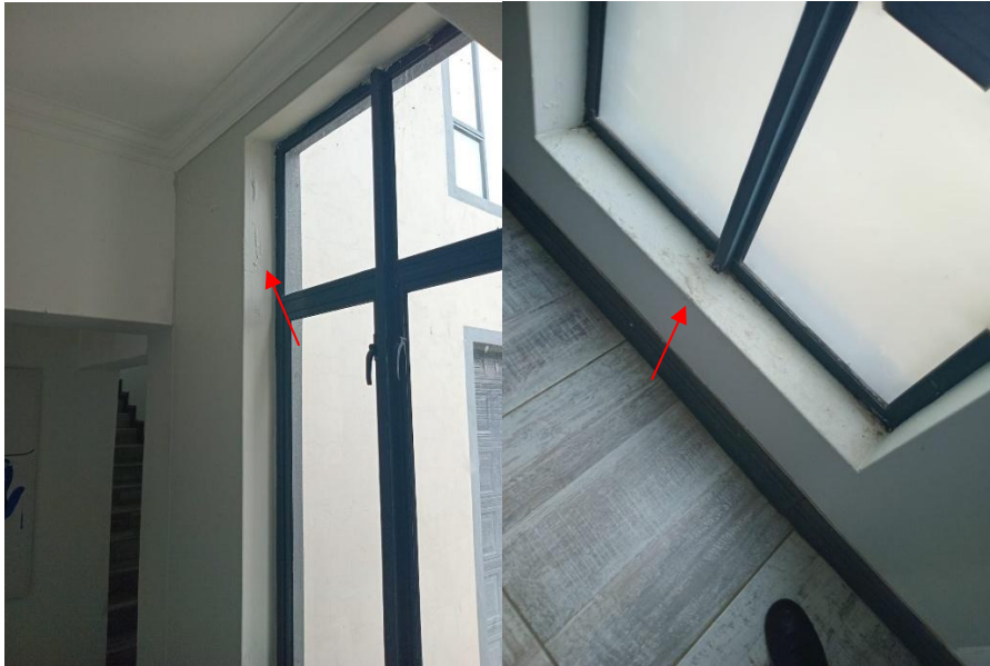
Figure 10: Window at Entrance Foyer
