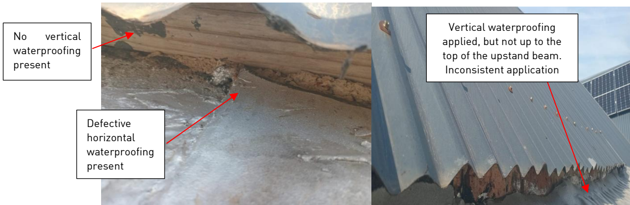
Figure 11: Vertical and Horizontal Water proofing
