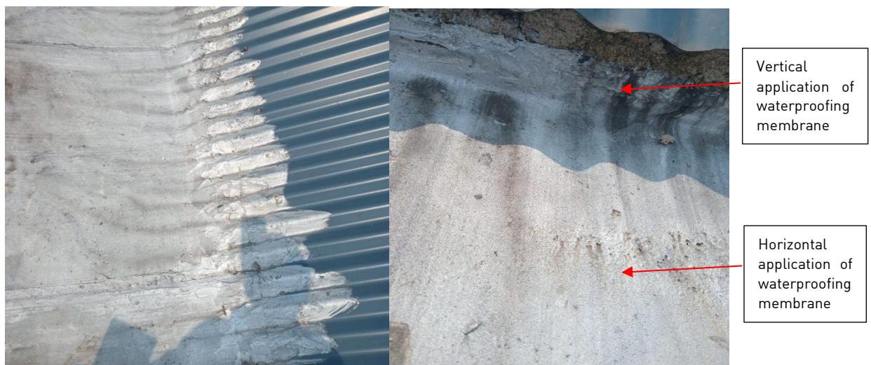
Figure 4: Edges of drainage slab 1
