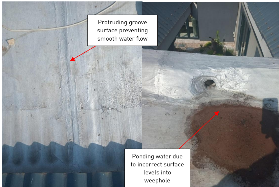
Figure 13: Concrete slab surfaces
